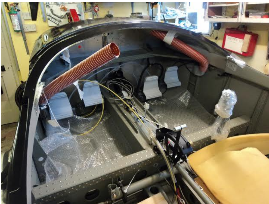
Looking worse than when I started!
